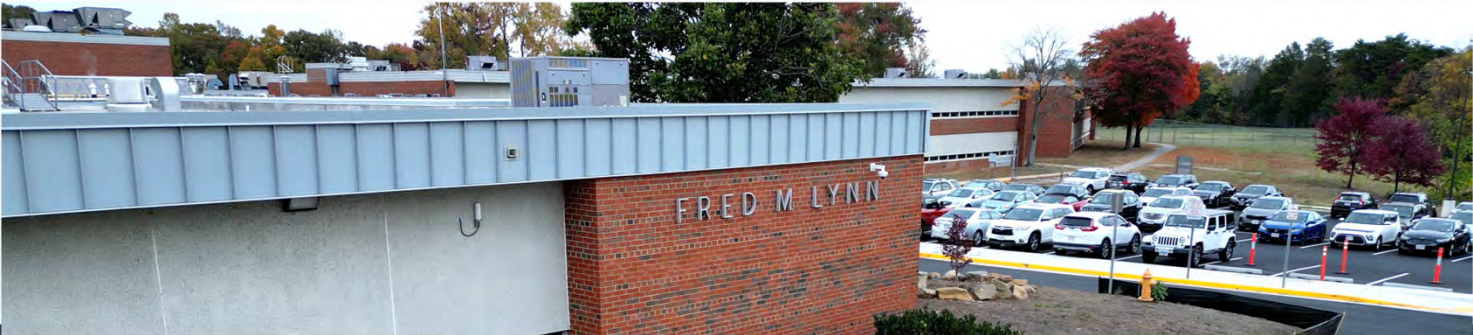
A project to renovate Fred M. Lynn Middle School.
